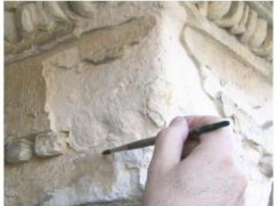
**Figure 13: Application of nanoparticles on degraded stones surface in Cà Granda, Milan, Italy. On the left, the untreated and powdery portion of Pietra D'Angera. On the right, application of consolidating nanodispersion by means of a brush.**
