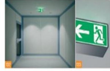
Escape sign luminaire for identifying escape route
