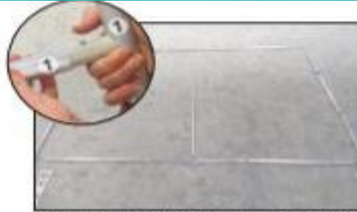
Align like numbers in sequence. Align #1 to #1 and #2 to #2 and so on.
