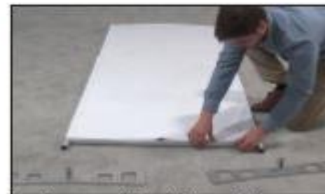
Continue attaching the liner with some tension.
