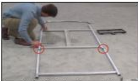
Insert BOTTOM of the frame until button locks engage.
