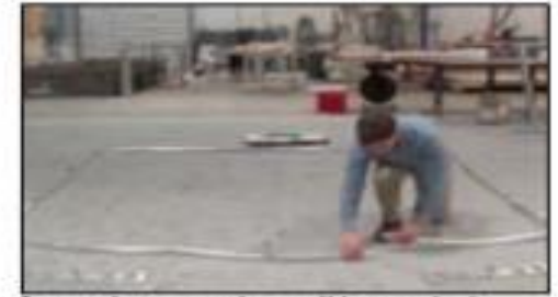
Insert the next tube until button lock engages.
