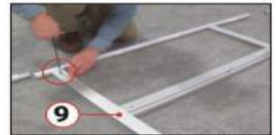
Insert part #9 into hole on the other side tube and secure CAM Lock using hex key.
