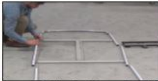
Connect the side tubes. Insert tube until button lock engages.
