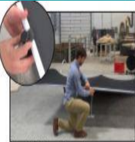
Attach lighting. Tighten clamp to secure lighting.
